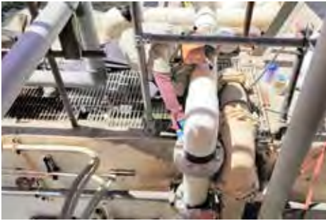
RSD Operations Staff Repairing Piping at the Treatment Plant.
