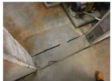
Electrical Room - f - large cracks opened in concrete fl...
