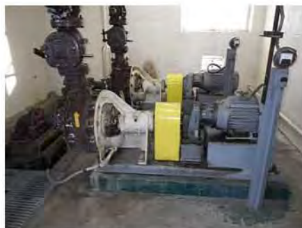
sludge recirculation pumps.jpg
