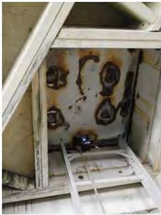
Heavily Corroded Access Hatch.jpg
