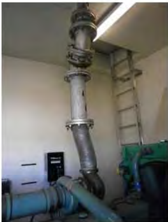
Influent Pump Station - a - generator exhaust connecti...
