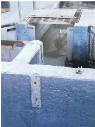
anchor stubs resulted in cracking.jpg
