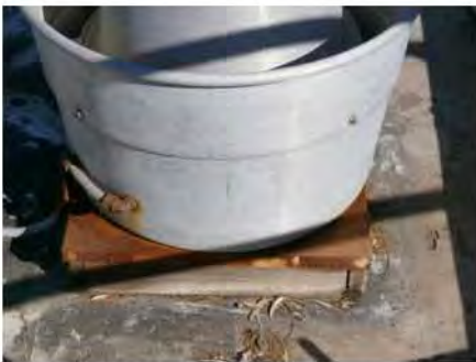
poor detailing for fan mounting curb and corroded flas...
