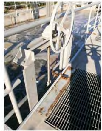
coverplates corroded with no support 2.jpg
