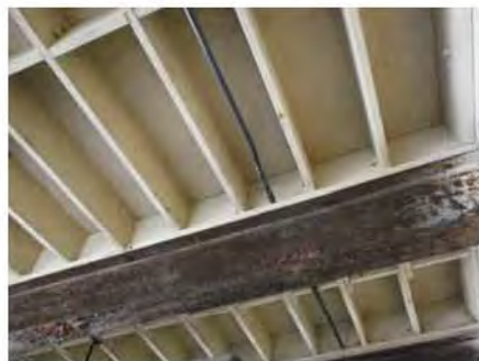
Roof Beam Corroded needs coating 1.jpg
