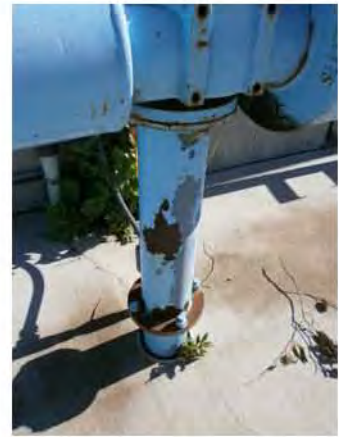
Corroded Pipe Support 2.jpg
