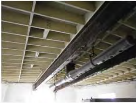
Roof Beam Corroded needs coating 3.jpg
