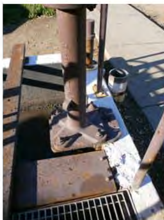
spalled concrete and corroded cover plates.jpg
