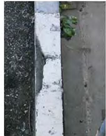
Site General - - Spalling of Curb.jpg
