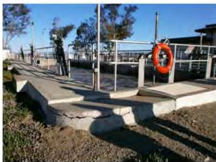
slab on grade walkway settlement.jpg
