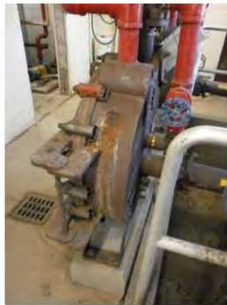
Electrical Room - b - corrosion on heat exchangers.jpg
