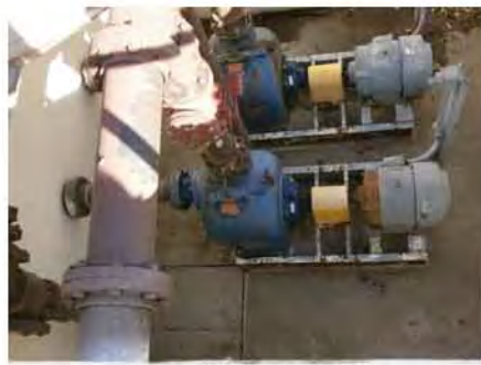
Heavily Corroded Pump Skid 2.jpg
