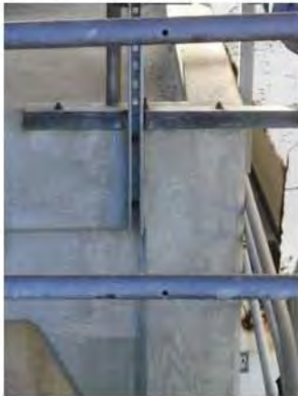
Dissimilar Metals Corrosion Uni strut Supports.jpg
