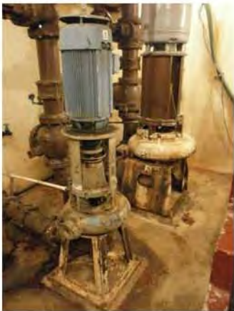
Influent Pump Station - d - heavily corroded pump sup...
