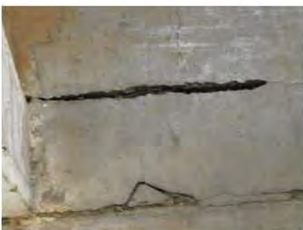
Electrical Room - g - large cracks opened in concrete f...
