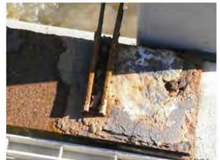
exposed rebar and spalled concrete at grating rebate.jpg...heavily corroded coverplates and instrument support.jpg
