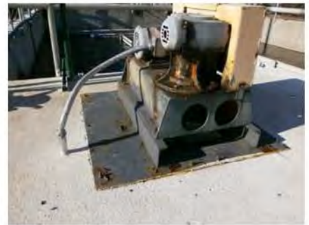
pump skid needs coating.jpg
