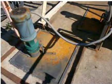
Influent Pump Station - i - heavily corroded opening co...
