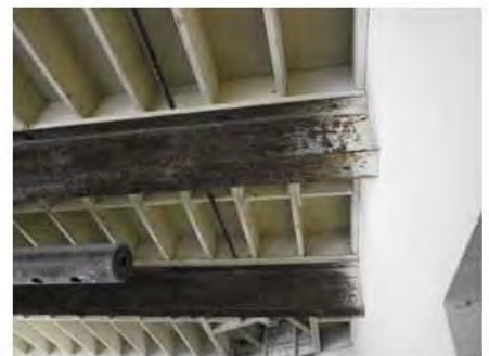
Roof Beam Corroded needs coating 2.jpg
