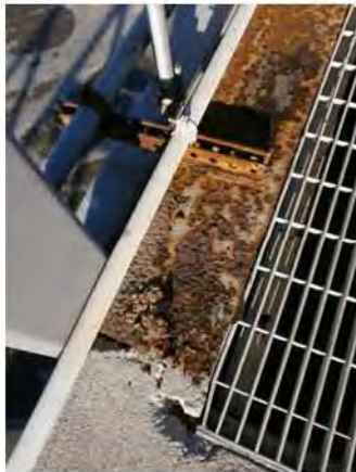
coverplates corroded with no support 3.jpg
