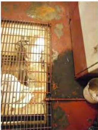
Influent Pump Station - g - spalled concrete at floor op...
