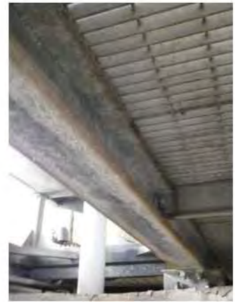
Heavily Corroded Mezzanine Support Beam 2.jpg
