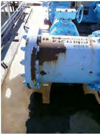
corroded pipe needs coating.jpg
