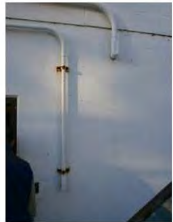
corroded unistrut pipe support.jpg
