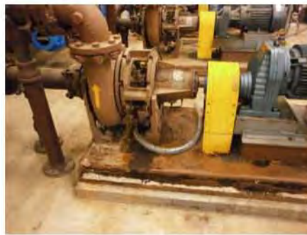
heavily corroded pump skids in effluent pump station.jpg
