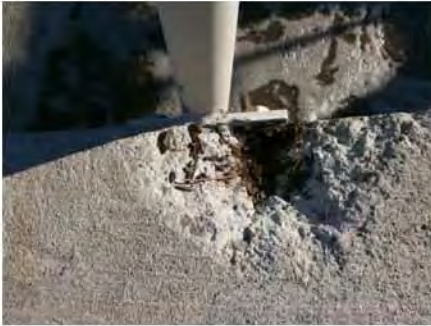
spalled concrete at guardrail attachment to concrete.jpg
