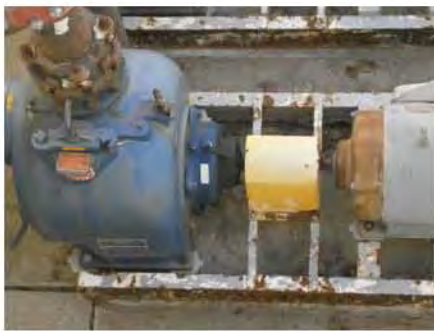
Heavily Corroded Pump Skid 1.jpg
