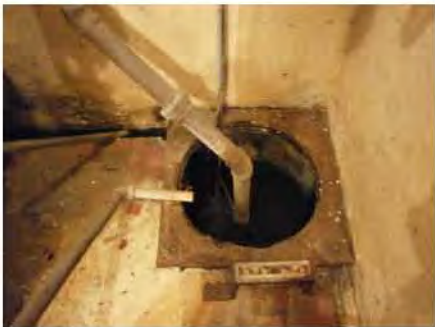
Influent Pump Station - f - heavily corroded sump cove...
