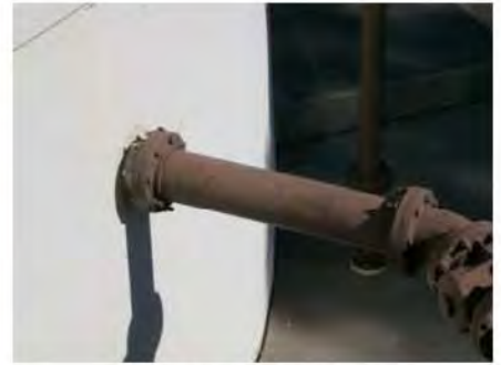
pipe flexibility required 2.jpg
