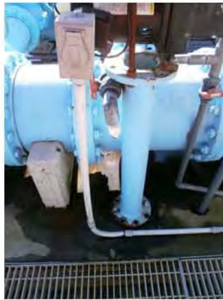
Corroded Pipe Support 1.jpg
