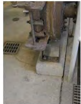
Electrical Room - c - corrosion on heat exchangers.jpg
