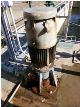
corroded pump support.jpg
