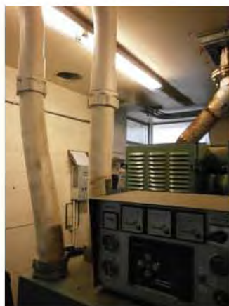
Electrical Room - h - flexible conduits at the generator....
