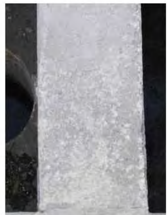
deteriorated concrete cover.jpg
