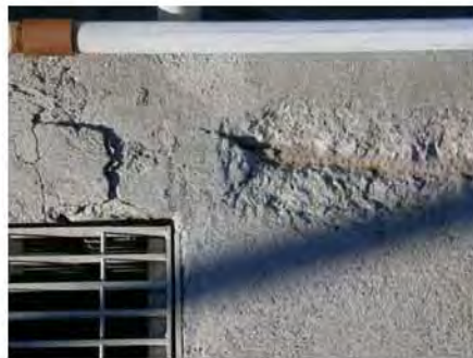
exposed rebar and spalled concrete at grating rebate.jpg...heavily corroded coverplates and instrument support.jpg
