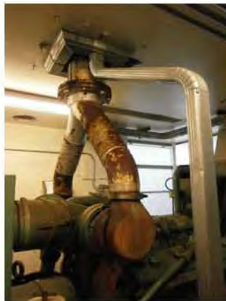
Electrical Room - k - generator exhaust connection.jpg
