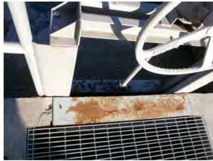
coverplates corroded with no support 1.jpg
