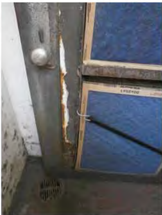
Influent Pump Station - h - acoustic door lining.jpg
