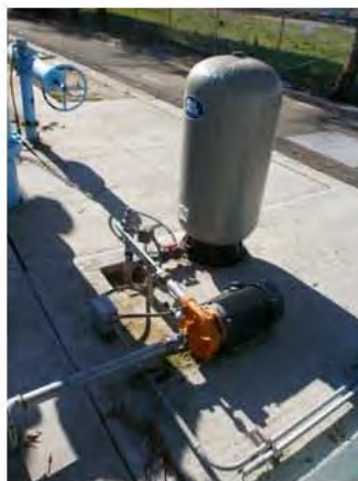
water surge tank unknown anchorage.jpg
