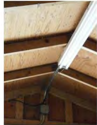
MCC Room - a - roof joists need blocking.jpg
