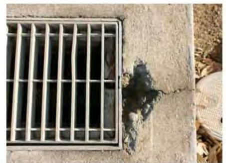
spalled concrete at grating rebate opening.jpg
