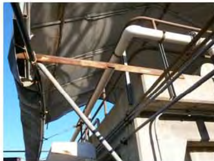
Minor Corrosion of canopy support .jpg
