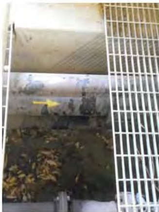
Electrical Room - d - coating of pipes needed.jpg
