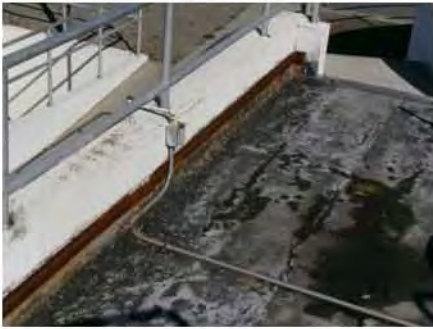
Deteriorated Flashing.jpg
