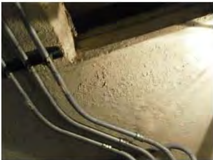
Influent Pump Station - c - roof leak and blistering of th...
