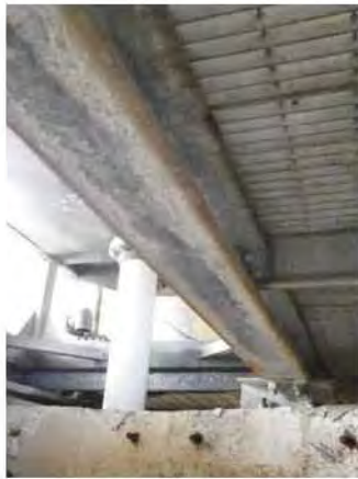
Heavily Corroded Mezzanine Support Beam 1.jpg
