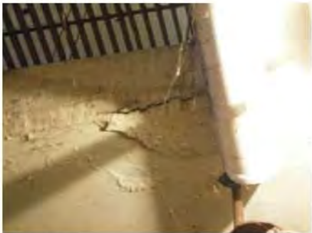
Influent Pump Station - e - concrete spalling at floor op...
