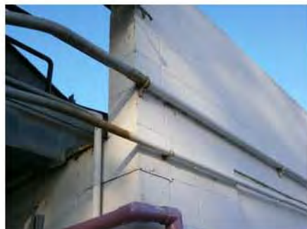
damaged masonry parapet + pipe corrosion.jpg
