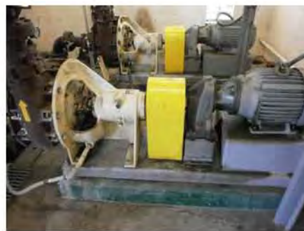
Electrical Room - e - no isolation for pumps.jpg
