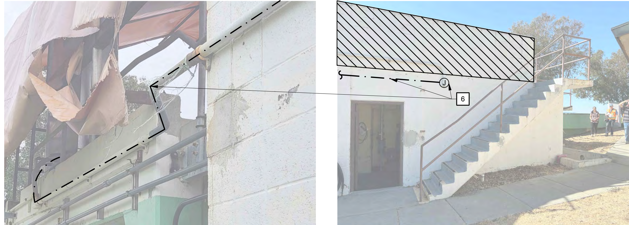
PHOTO - HEADWORKS STRUCTURE (4) SCALE: NO SCALE
