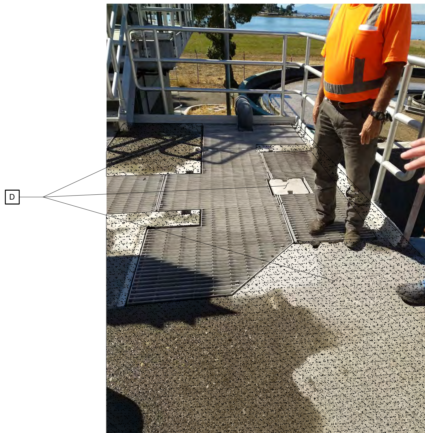
PHOTO - HEADWORKS STRUCTURE 5 SCALE: NO SCALE M203
