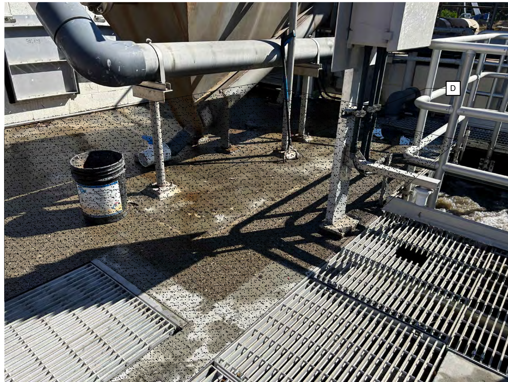
PHOTO - HEADWORKS STRUCTURE 3 SCALE: NO SCALE M203
