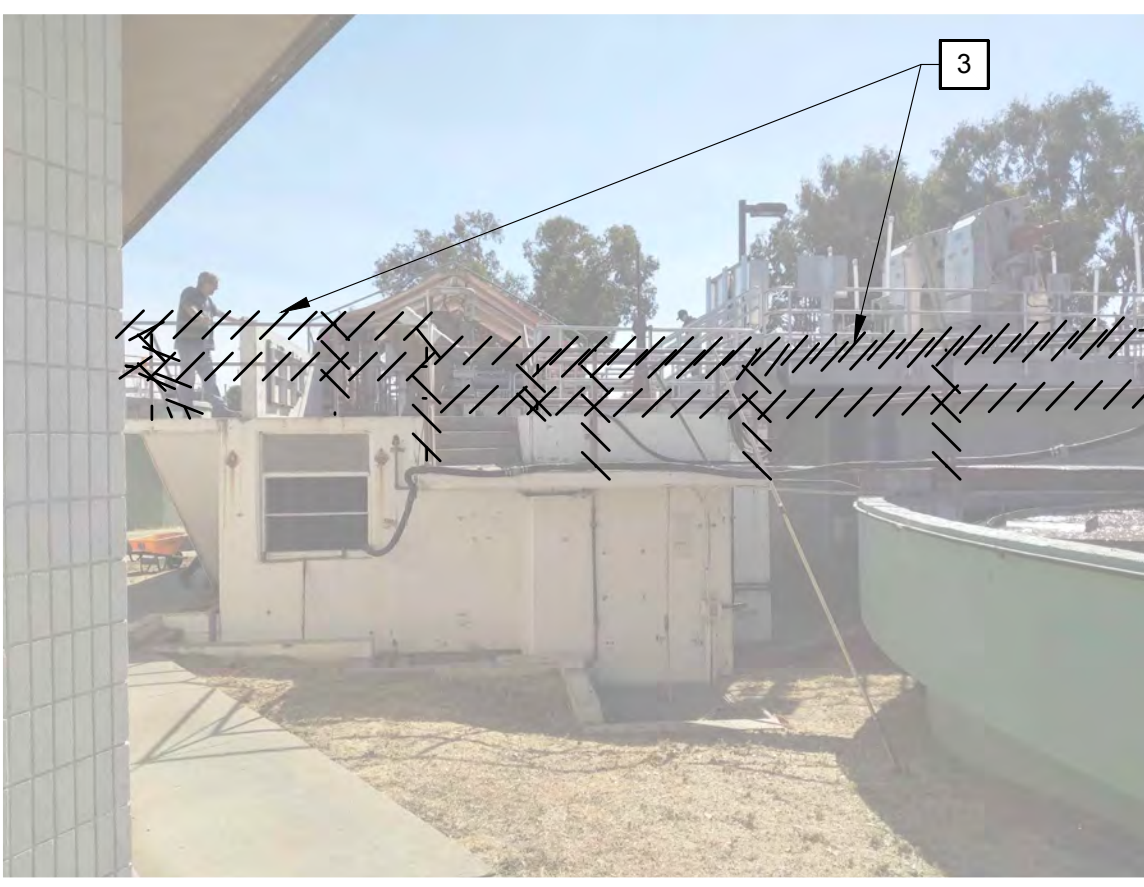
PHOTO - HEADWORKS STRUCTURE SCALE: NO SCALE
