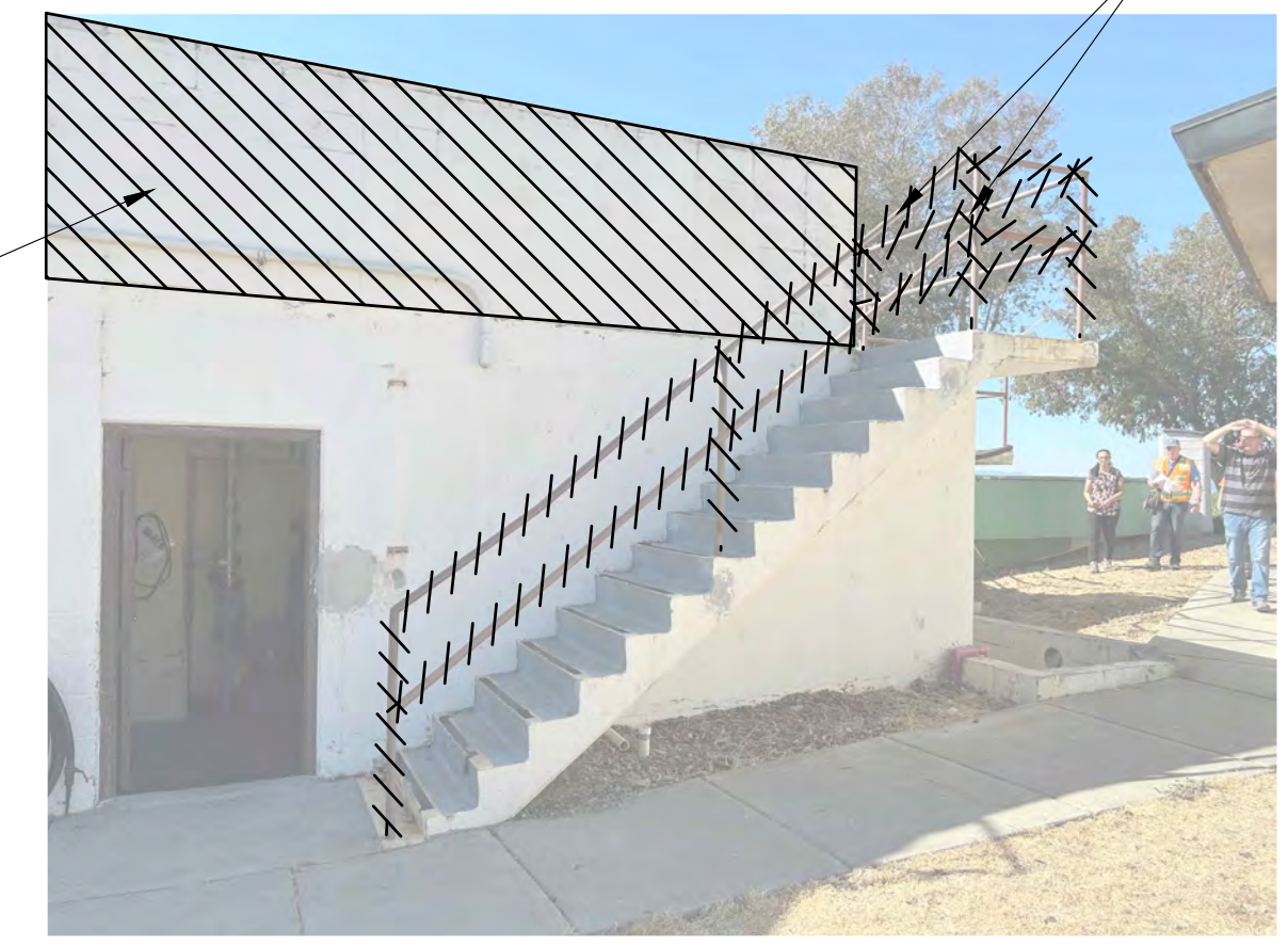
PHOTO - HEADWORKS STRUCTURE SCALE: NO SCALE
