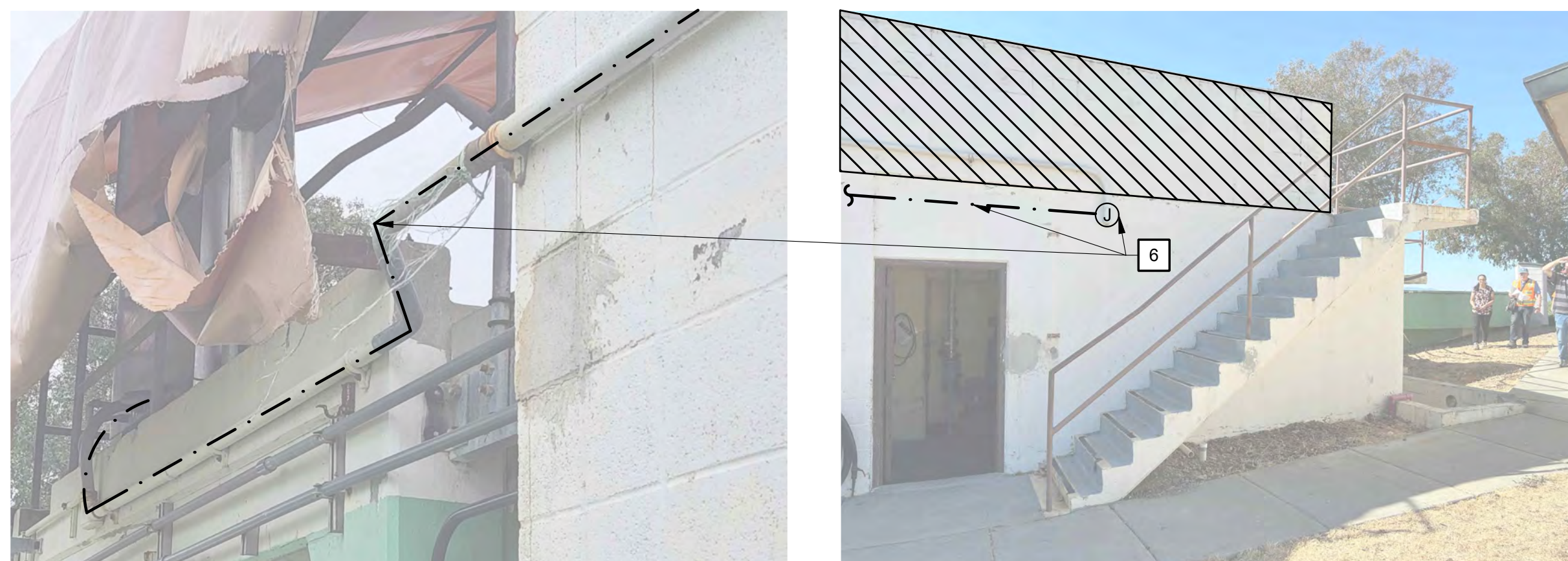
PHOTO - HEADWORKS STRUCTURE (4) SCALE: NO SCALE
