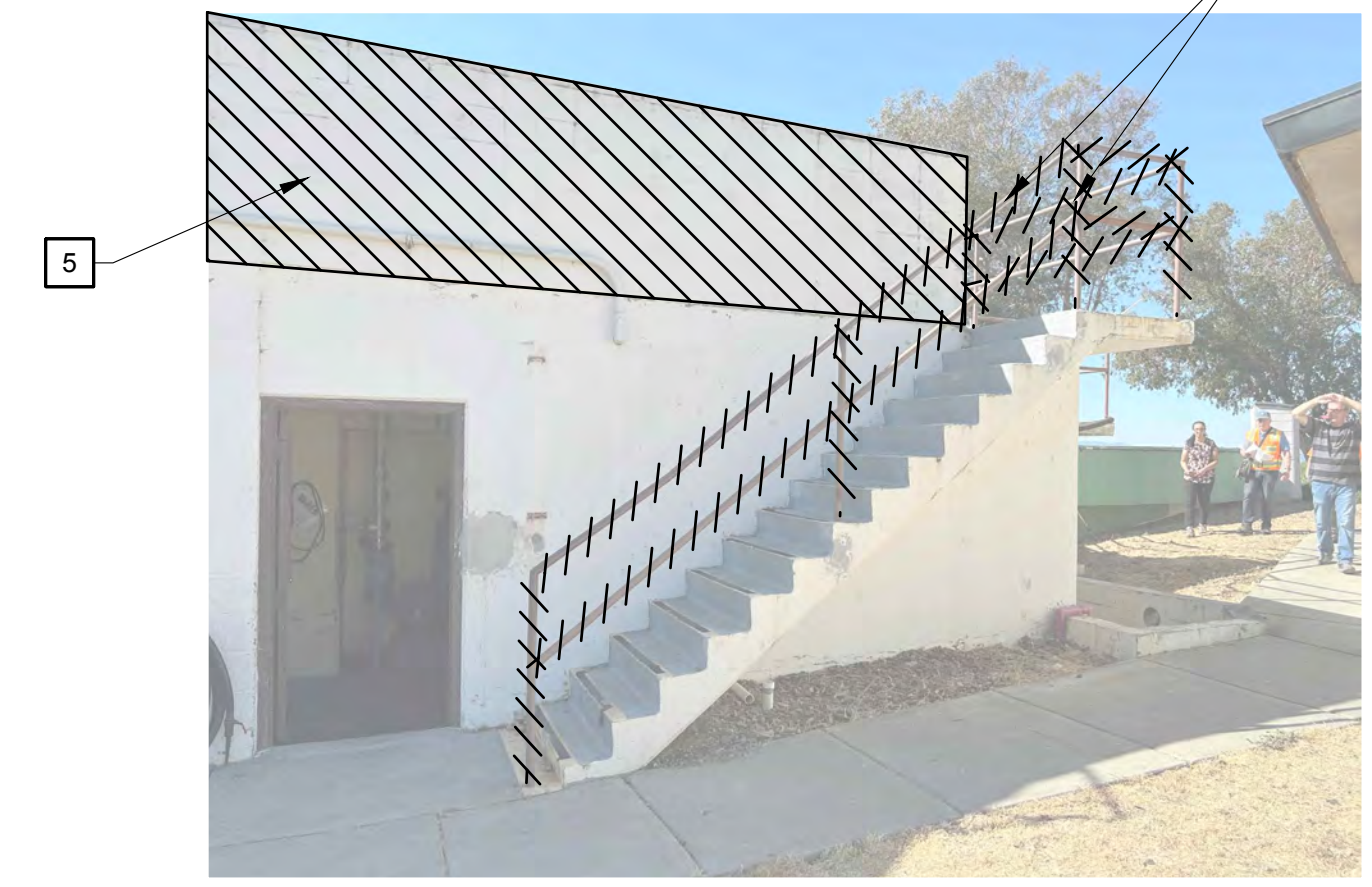
PHOTO - HEADWORKS STRUCTURE SCALE: NO SCALE
