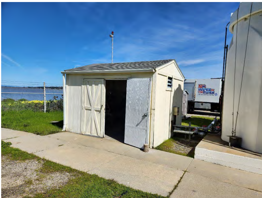
Chemical Feed Building
