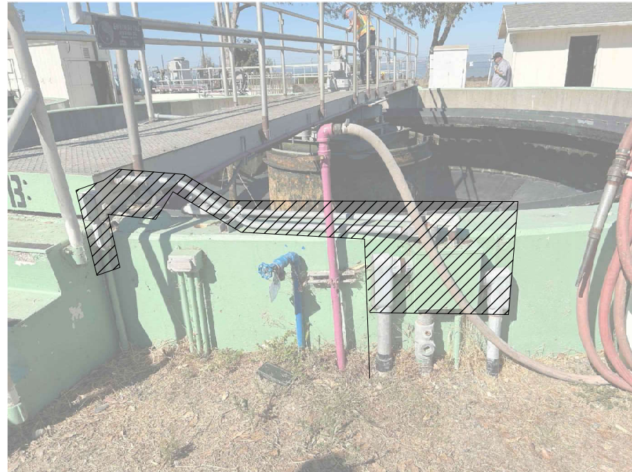
PHOTO - SECONDARY CLARIFIER ① SCALE: NO SCALE
