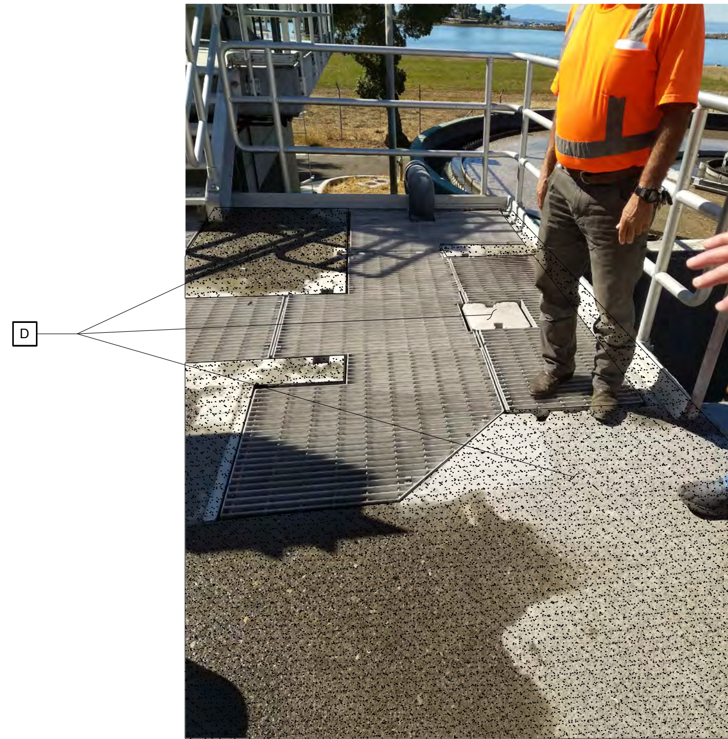
PHOTO - HEADWORKS STRUCTURE 5 SCALE: NO SCALE M203
