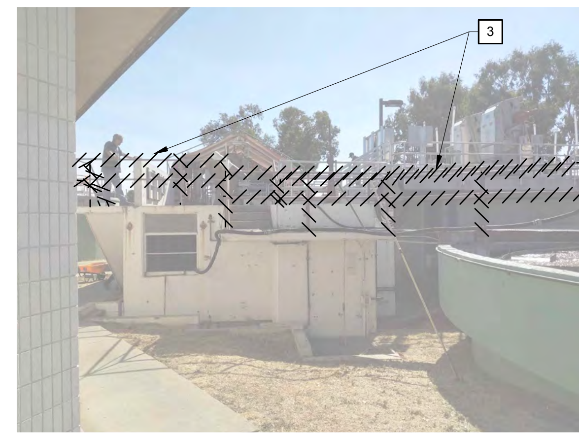
PHOTO - HEADWORKS STRUCTURE SCALE: NO SCALE
