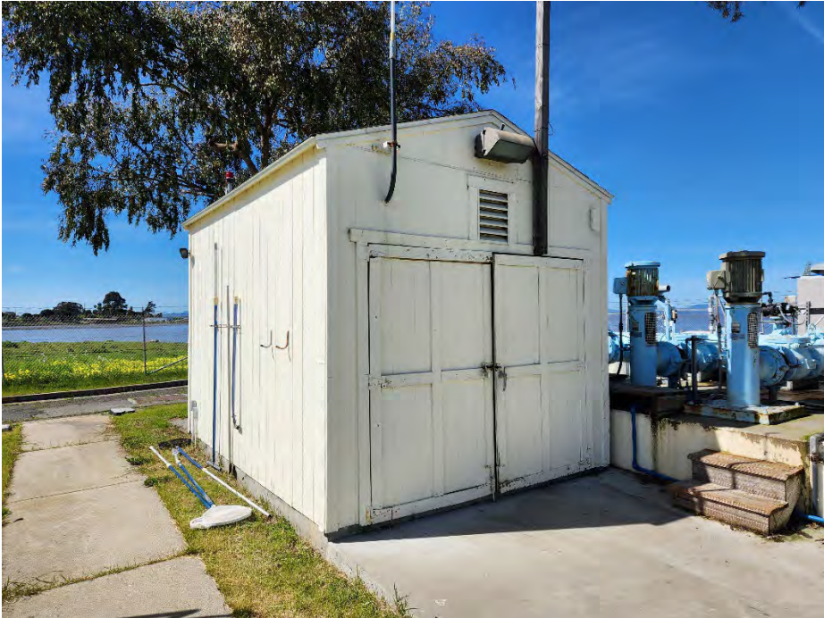
Effluent Pump Station Building
